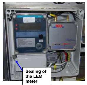
Detailed view of an EMU, showing sealing of the LEM meter.
